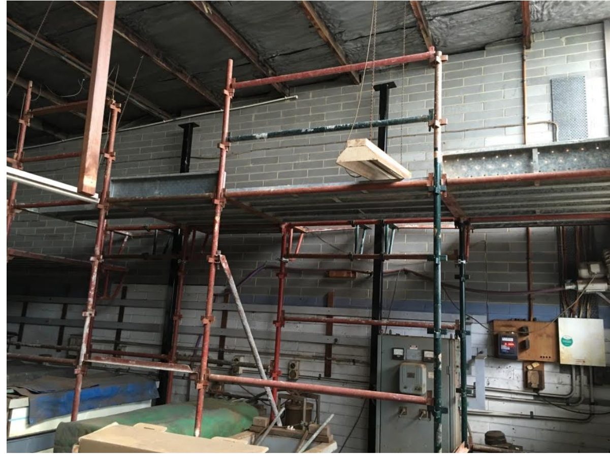
Fire Separation Works
