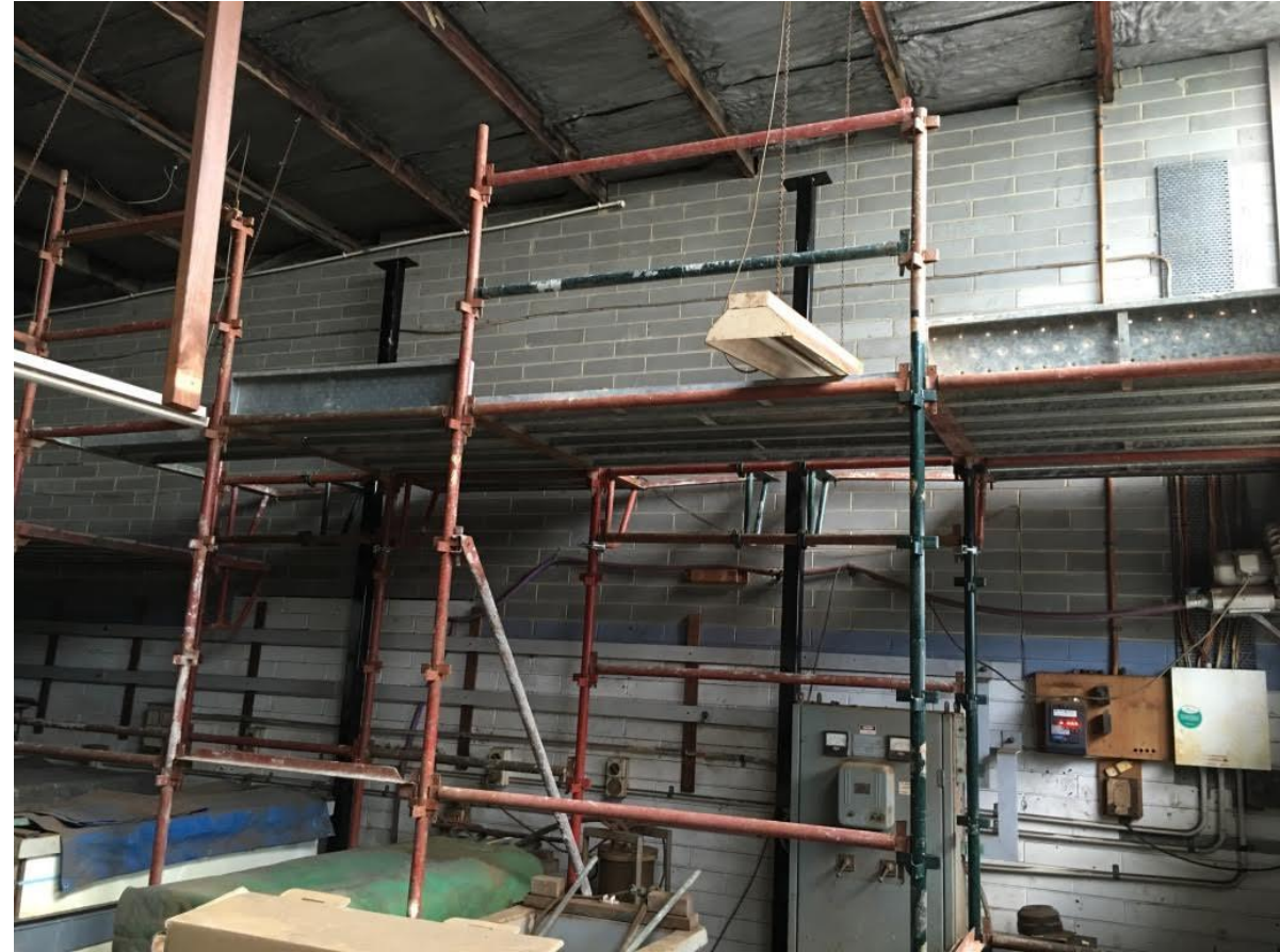
Fire Separation Works
