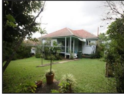
Rear of House & Back Yard
