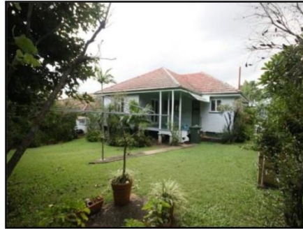
Rear of House & Back Yard
